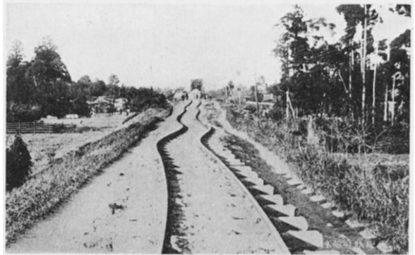
FIG. 5. Buckling of rails on the approach to the Kisagawa railroad bridge after the great Japan earthquake of 1891.
